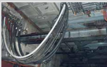
Heated hose (nominal diameter 50) for connecting storage tank and extinguishing water distribution system. Function: Protection against freezing (+ 5°C) outdoors. Material-transfer hose made of polyethylene
