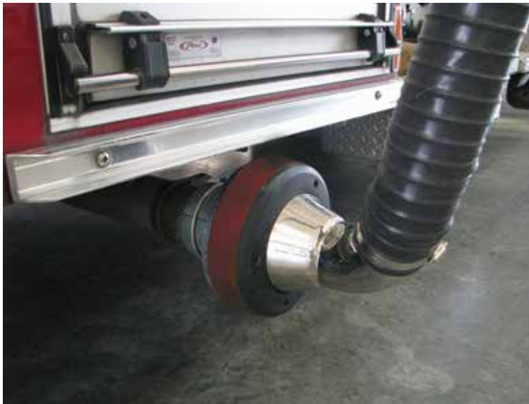
Rigid, reinforced 2-ft section of high-temp Fire Flex® dual temperature hose, below the safety disconnect, enables the firefighter to place the hose collection nozzle onto the tailpipe without bending over.
